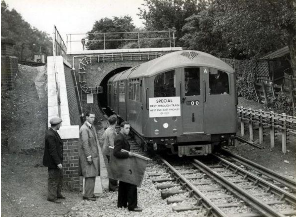
East Finley underground train in 1939
